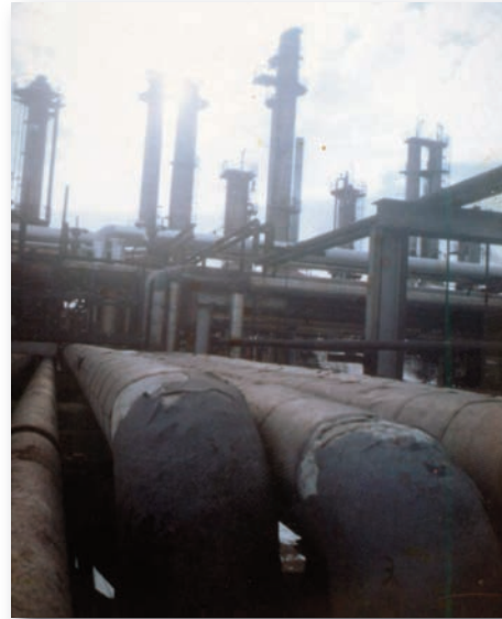
Pictured above: Ashland Oil refinery in Tonawanda, New York, as it appeared in the late 1960s. As seen in the picture above, asbestos insulation covered miles of pipeline at this facility.
