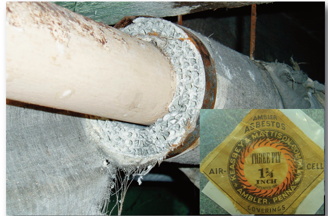
Pictured above, cross section of Aircell, asbestos pipe insulation.
