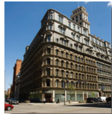
The Historic Powers Building
